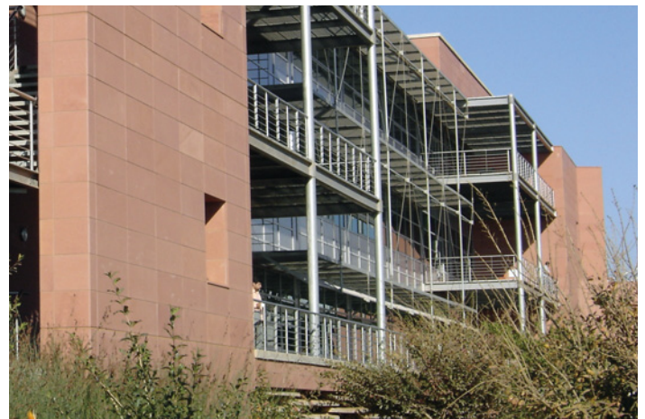
The above photos show varying views on the MTN Headquarters, Johannesburg, South Africa, where hot dip galvanized steel was used architecturally.
