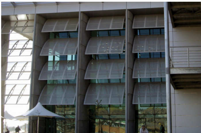
The above photos show varying views on the MTN Headquarters, Johannesburg, South Africa, where hot dip galvanized steel was used architecturally.
