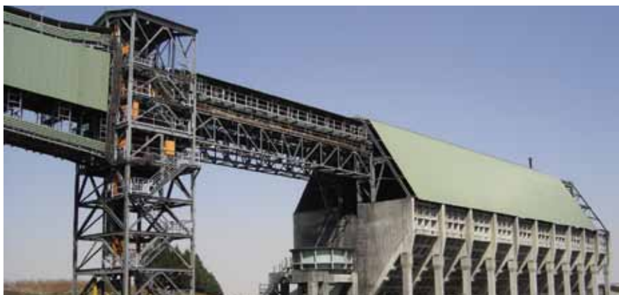
Photo 36: The transfer tower and hopper.
