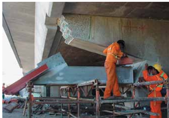
Photo 4: Positive anchoring of widened pier elements to the existing by using GEWI post tensioned anchors.
