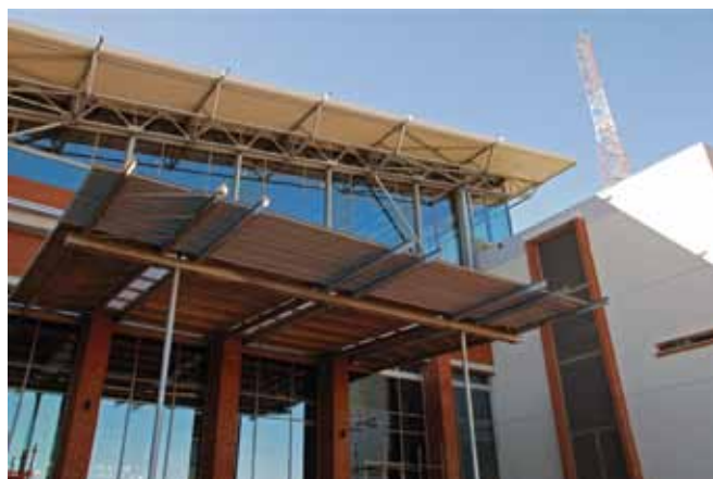
Photo 3: Gate house and hot dip galvanized steel canopy.
