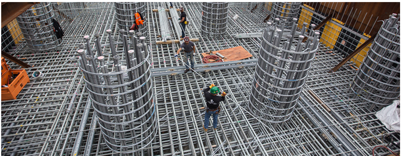
Using hot dip galvanized rebar in a structure prior to pouring concrete – galvanised rebar extends the life of bridges, waterworks structures and all manner of municipal concrete structures
