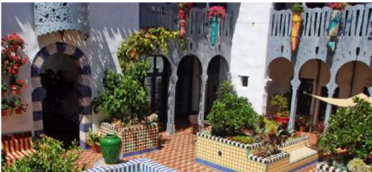
Beautiful integration of hot dip galvanized steel with coloured coatings & tiles
