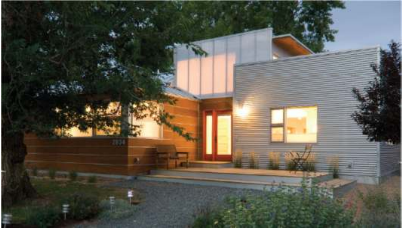
Use of continuously galvanized sheeting as building cladding – in this case a galvalume cladding
